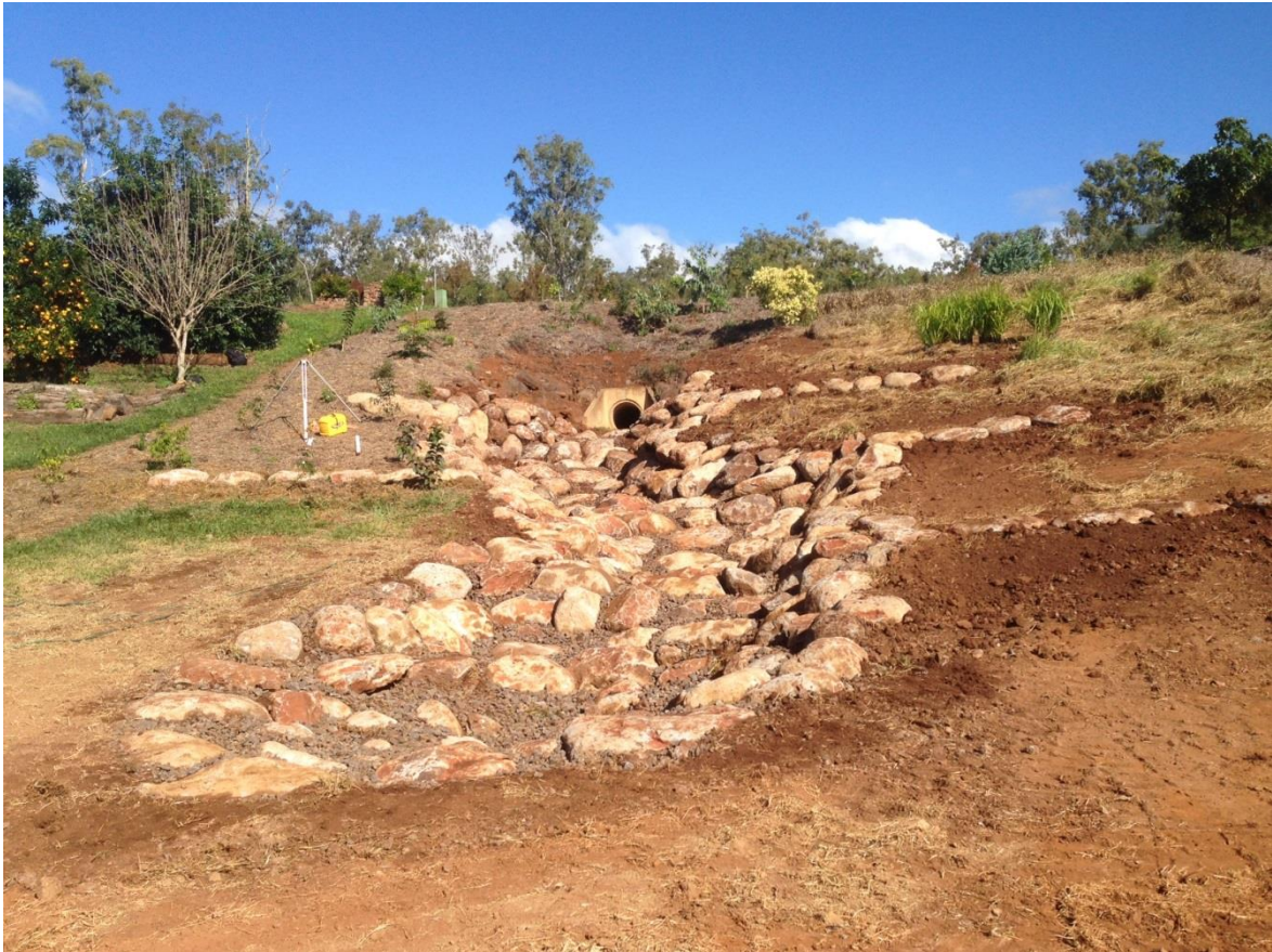
Figure 2. Rangeview Culvert Upgrade
