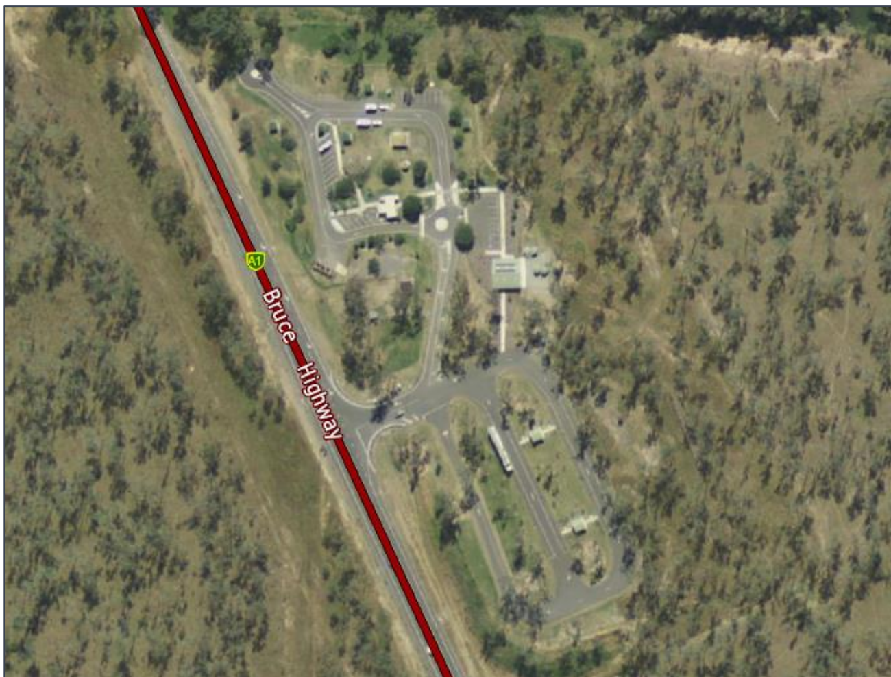
Figure 4: Aerial photo of Waverley Creek Rest Area (Source: Queensland Globe, 2018)
