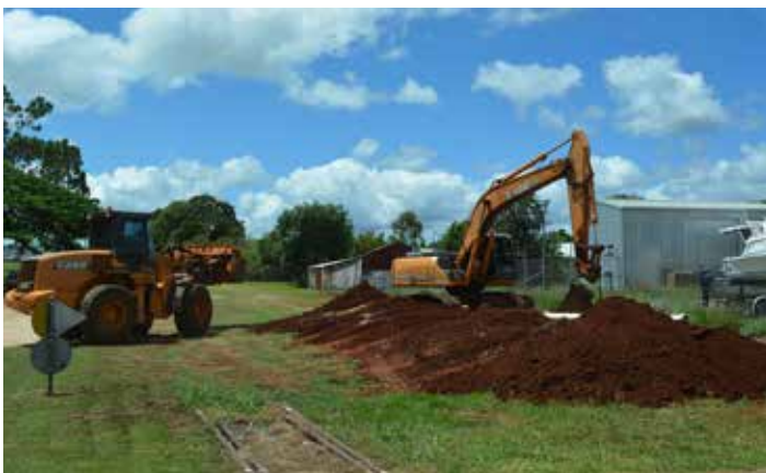
Commencement of works – Atherton Rail Trail, Atherton
