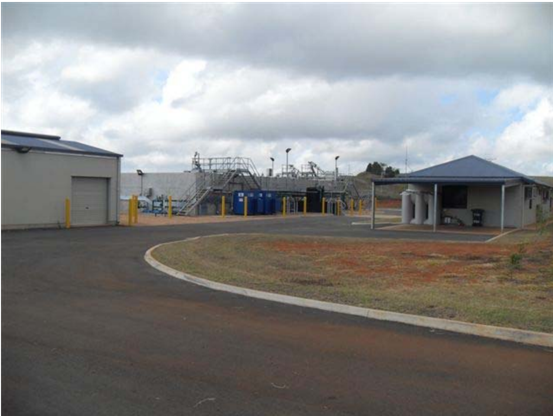
Figure 3: Malanda wastewater treatment plant installation
