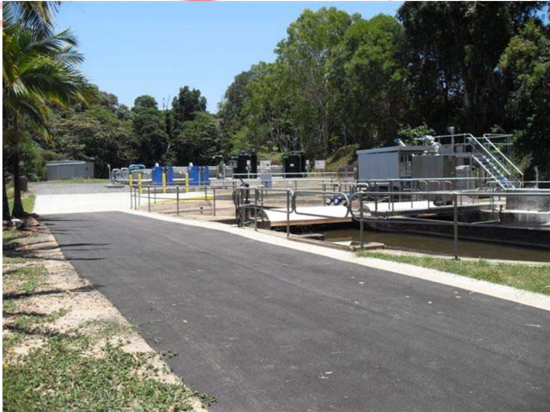
Figure 2: Kuranda wastewater treatment plant upgrade
