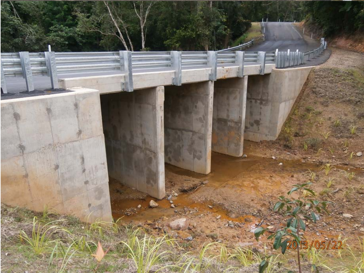
Jum Rum Creek Bridge, Fallon Road, Kuranda
