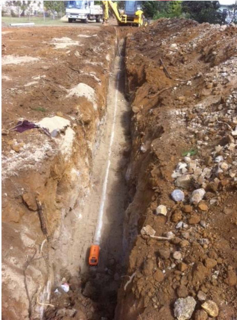
Figure 1: Mclver Road Mareeba sewer main installation
